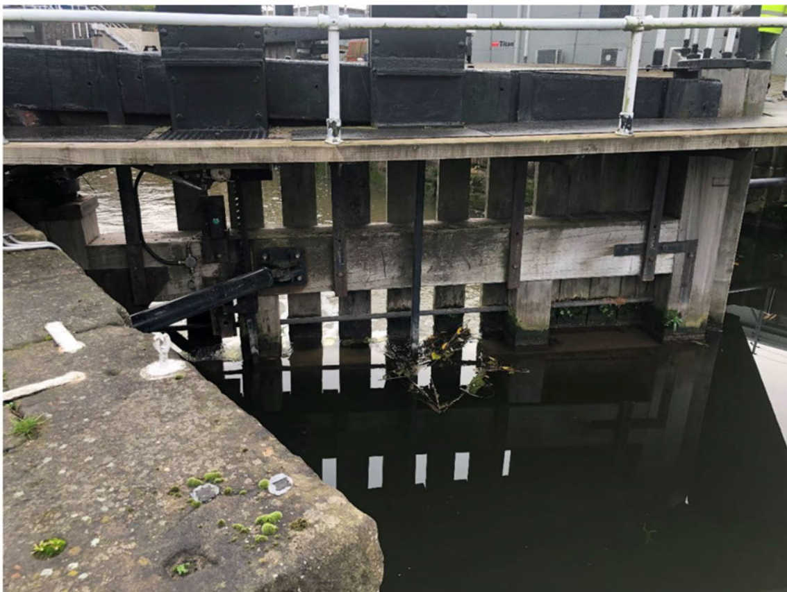
Figure 4 - Upstream face of the top lock gates to be modified at Keadby Lock (image Arcadis 2022)
